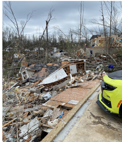
Damage near Newnan (Coweta County), Georgia Source: NWS Atlanta
