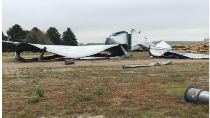
Straight-line wind damage in eastern Colorado
