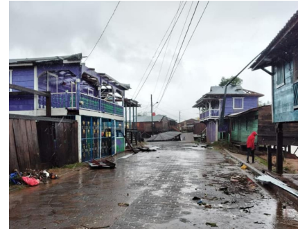
Damage in Prinzipolka (Nicaragua) Source: SINAPRED
