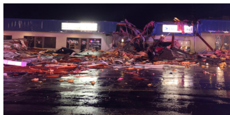
Osage Beach strip mall damage (Missouri) Source: Missouri State Highway Patrol
