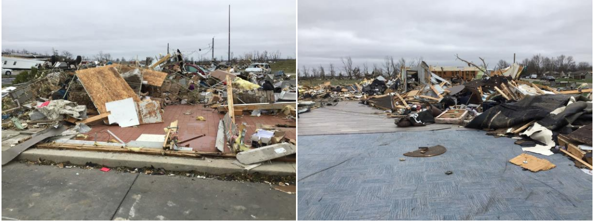
EF-3 Tornado Damage in Winchester, Indiana
