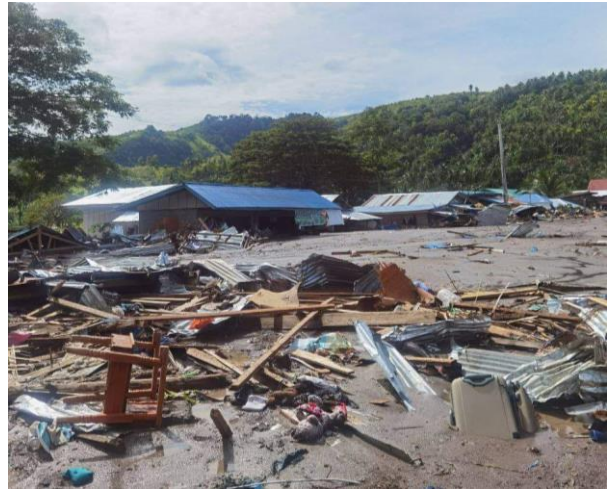
Flooding and landslides damages in Maguindanao Province
