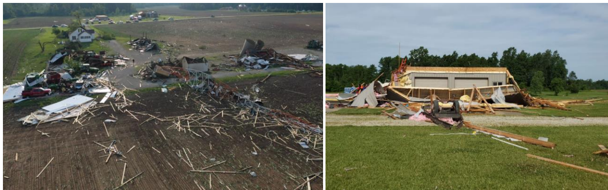
Tornado damage in Jay County, Indiana from June 18
