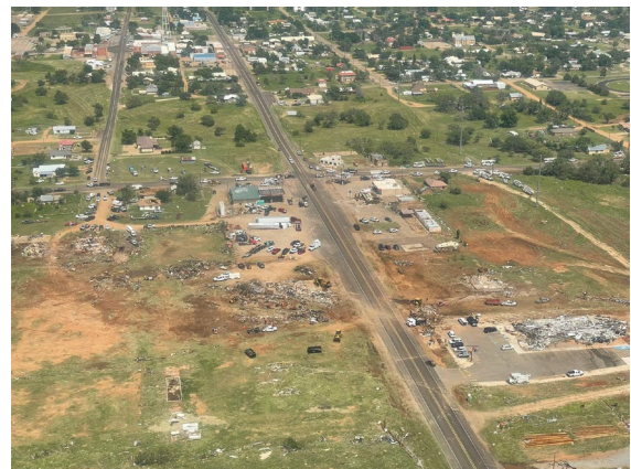
Tornado damage in Matador
