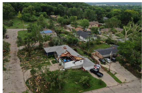
Wind damage in Riley County, Kansas Source: Riley County Emergency Management
