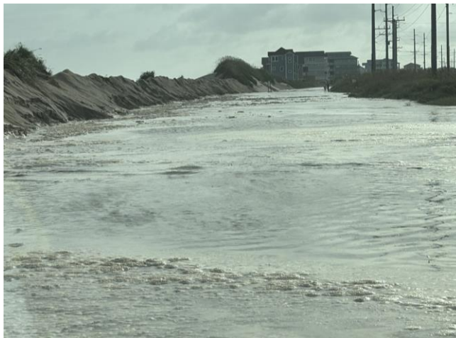
Coastal flooding and erosion in North Carolina Outer Banks
