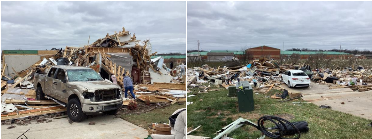
Tornado damage in Clarksville, Tennessee
