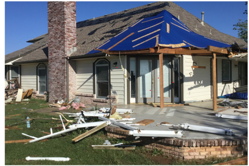
Tornado damage near Coweta, Oklahoma
