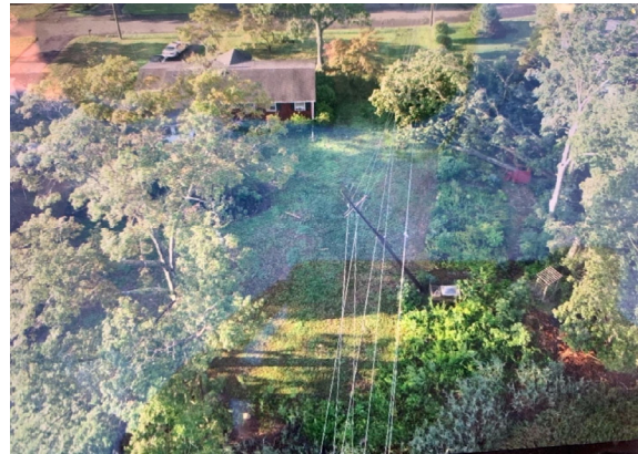
Storm impacts in Branford, CT. Source: Eversource CT
