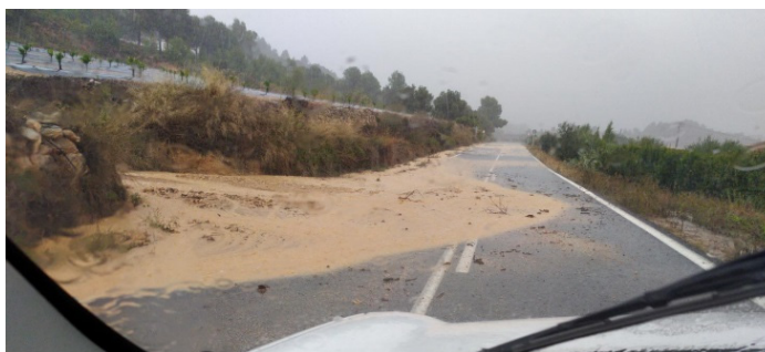
Washout and erosion damage on agriculture Source: Provincial Council of Valencia
