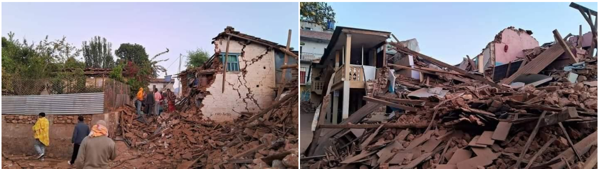
Structural damage in Jajarkot District
