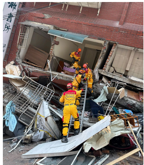
Earthquake damage in Hualien City Source: CECC
