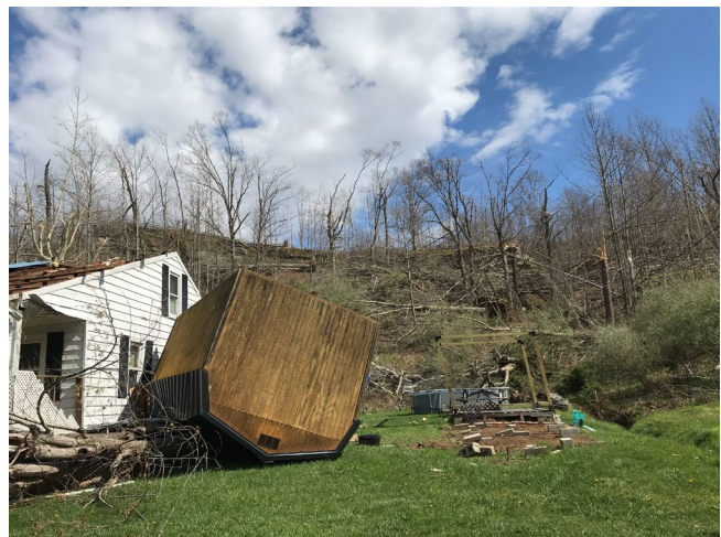
Tornado damage in Kentucky
