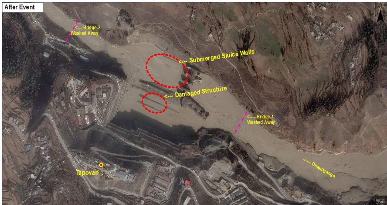
Damage caused by the GLOF activity on February 7
