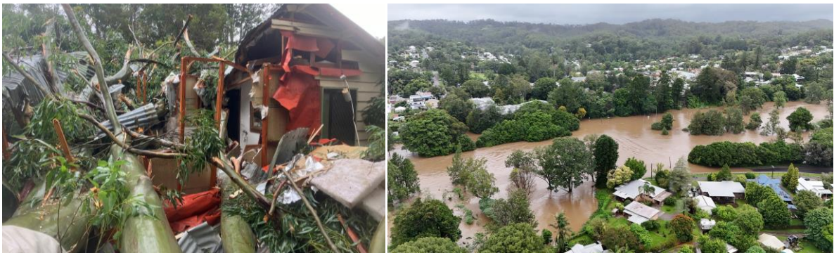
Flooding damage from Cyclone Alfred in QLD (left) and NSW (right) Source: Queensland FD (left), New South Wales SES (right)
