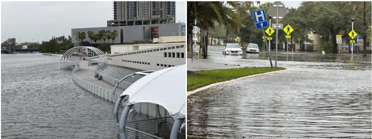
Flooding in Tampa, Florida Source: City of Tampa
