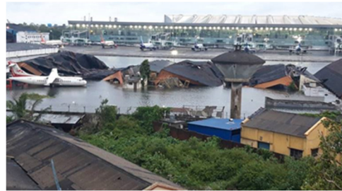
Flooding at Kolkata Airport (Source: Press Trust of India)
