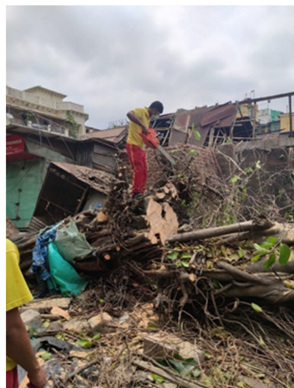
Source: Odisha State Disaster Management Agency
