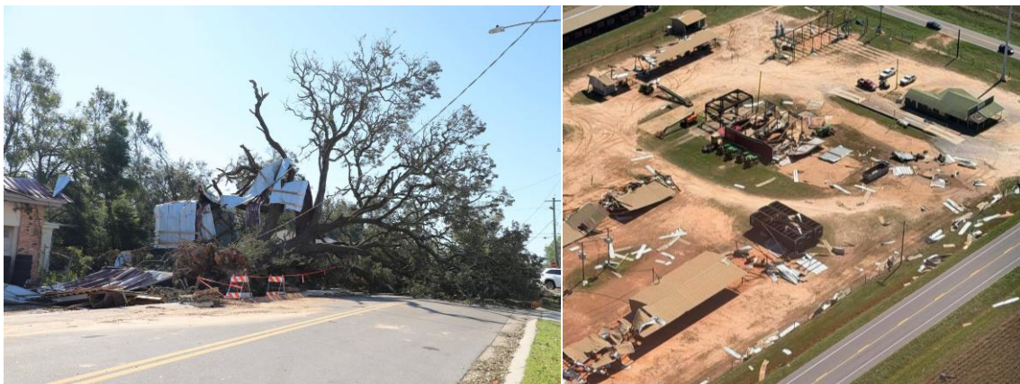
Hurricane Isaias wind damage in Escambia (left) and Santa Rosa (right) counties Source: Escambia County; Santa Rosa County Sheriff Office
