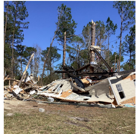
Tornado damage in Brantley County, Georgia
