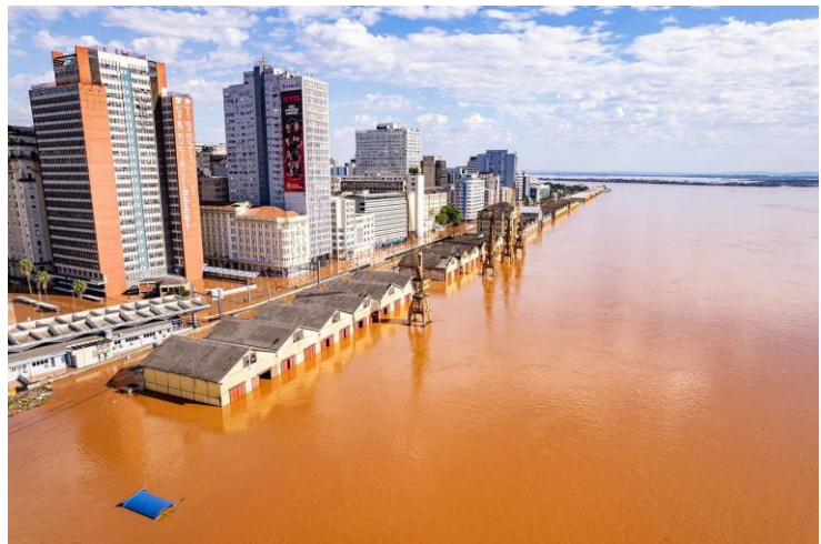
Flooding in Porto Alegre
