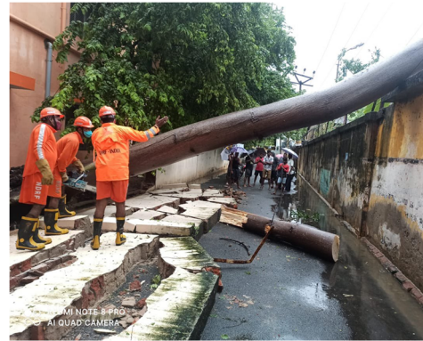
Damage Caused by TC Nivar in Tamil Nadu Source: NDRF, India
