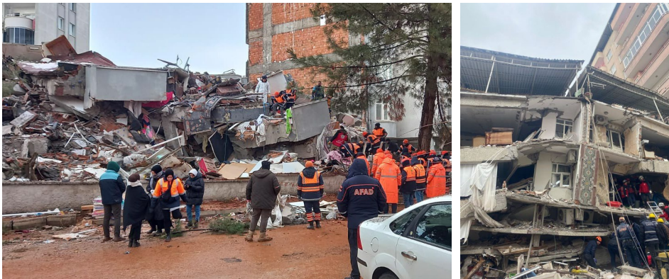
Earthquake damage in cities of Gaziantep (left) and Diyarbakir (right)
