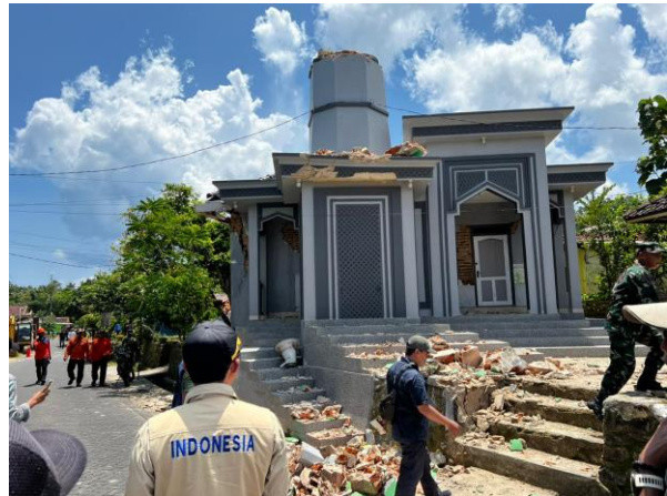
Damage in Bawean Island, Gresik Regency
