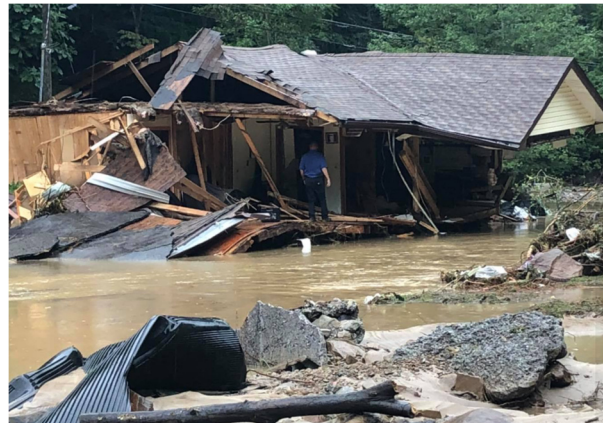
Flooding in Hurley, Virginia Source: Roanoke Fire-EMS
