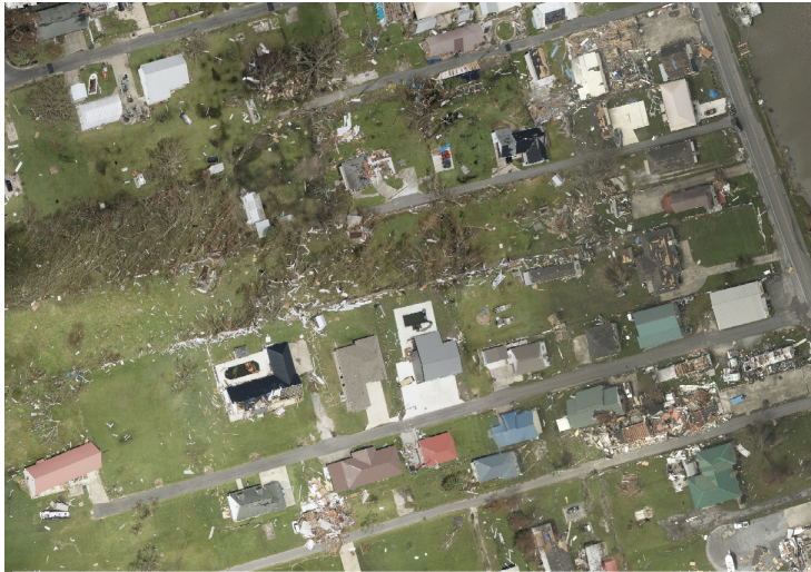
Wind damage to homes and timber in Golden Meadow, LA Source: NOAA
