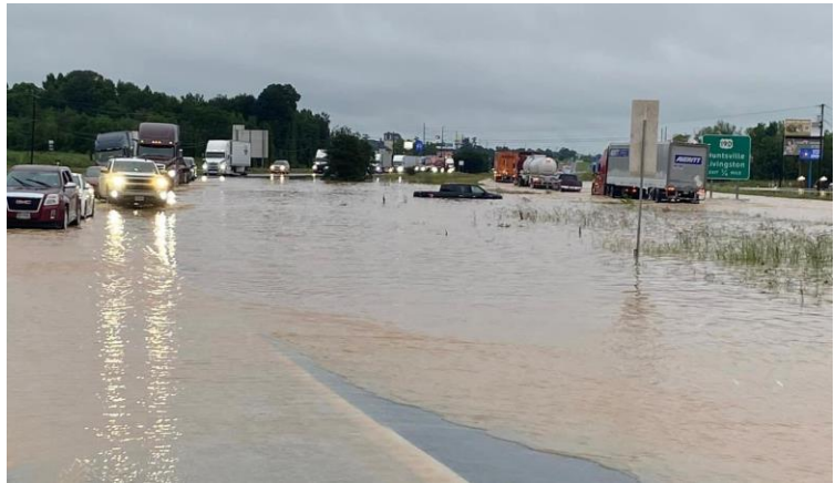
Flooding in Polk County, Texas
