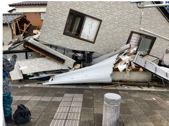
Earthquake damage in Wajima Source: Ministry of Defense
