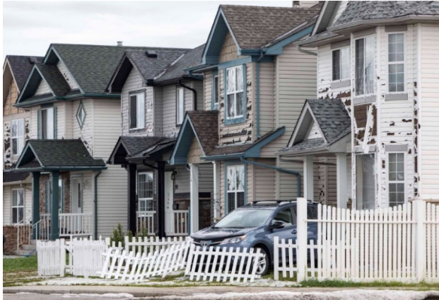
Damaged homes from Calgary hailstorm. Source: City of Calgary
