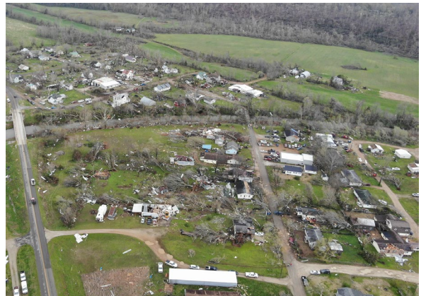
Tornado damage in Bollinger County, Missouri
