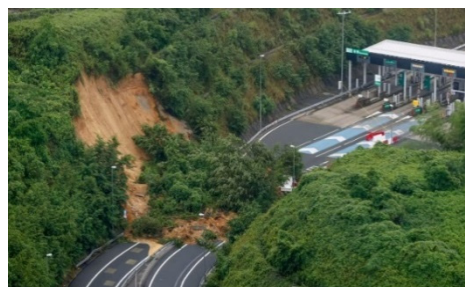
Landslide in Kyoto (Source: AP)
