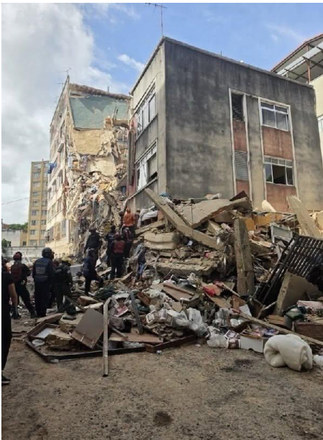
Collapsed buildings in Caracas.
