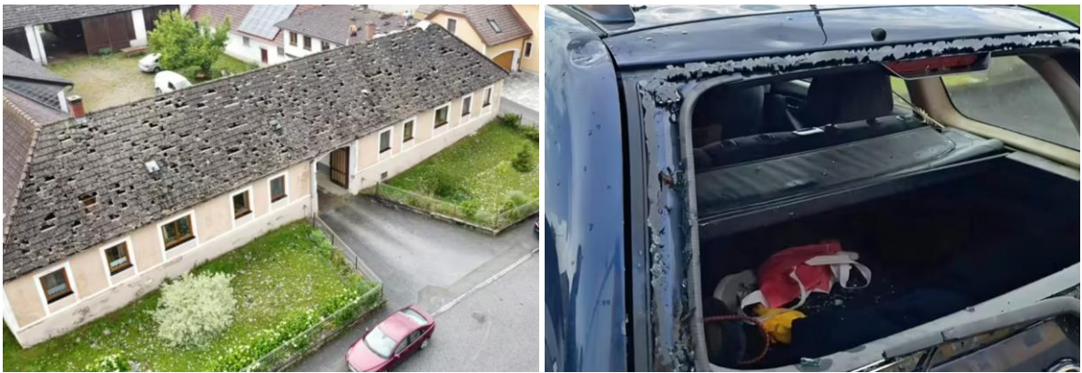
Hail damage in Waidhofen an der Thaya, northern Austria
