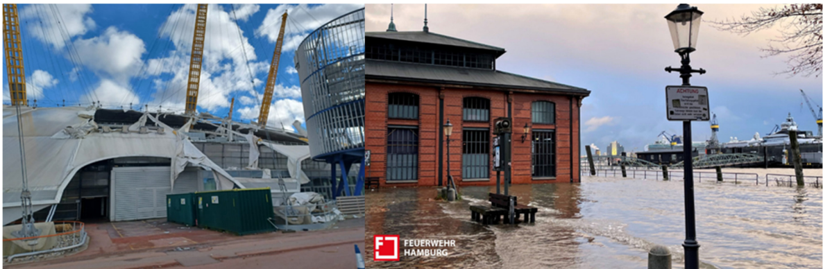
Damage to roof of O2 Arena in the U.K.
