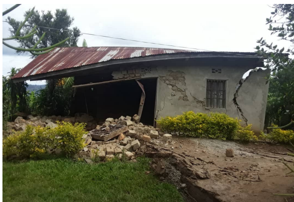
Source: Nyamasheke district, Rwanda
