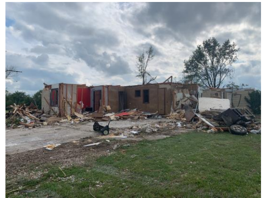
Tornado damage in Baring, Missouri
